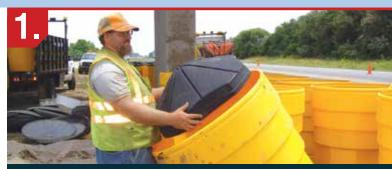
Lean the barrel inward. Hold the Insert, cone-shaped side face up, with both hands.
