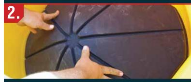
CrashGard Insert is a square-sided piece. Make sure the configuration of the Insert matches the configuration of the barrel shelf upon which it rests. Drop the Insert into position.
