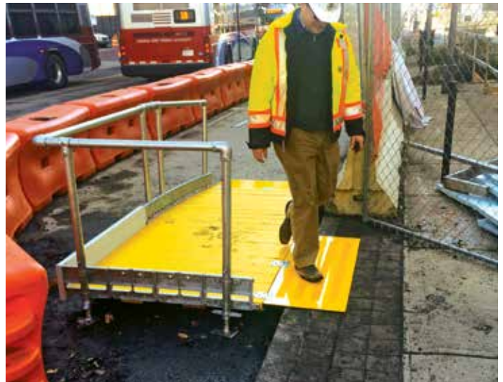
BoardWalk Ramp shown parallel to curb, with Platform.
